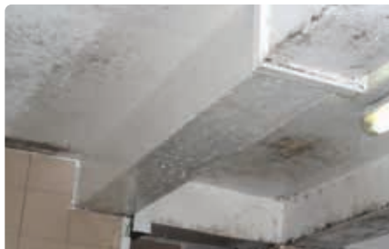
During application and cleaning with BioProtect™ Industrial Treatment
